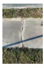
The photo to the left shows a joint where concrete has been chipped away from the joint. It can & should be filled instead of replaced with new concrete. We do not provide this type of work because most of our clients have maintenance staff that can do it less expensively on their own with materials purchased at local hardware stores.
