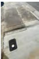
The photo to the left shows an area of sidewalk that should be replaced with new concrete. The surface is spalled, and it is too uneven for a repair. Because we do not provide concrete construction services, this is not work that we can provide. It will require a general contractor.
