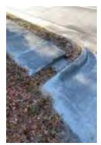
The photo to the left shows a driveway apron where sidewalk is missing, and where a ramp is needed to replace the curb in the driveway apron. Because we do not provide concrete construction services, this is not work that we can provide. It will require a general contractor.
