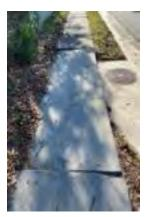
The photo to the left shows displacements that are too big to be repaired. The displacement is well over 2" high. Cutting away the high concrete will leave a slab that is too thin and susceptible to breaking. This piece
