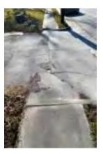
The photo to the left shows a driveway apron/crosswalk that should be improved. It is too broken and uneven. Because we do not provide concrete construction services, this is not work that we can provide. It will require a general contractor.
